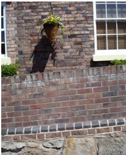
I4b. Brick wall built along incline
