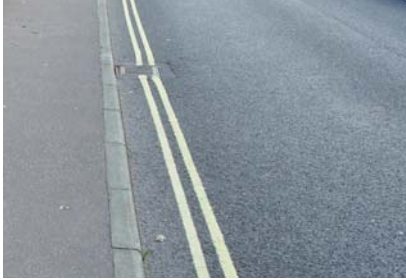
5a. Drainage channel within blacktop road
