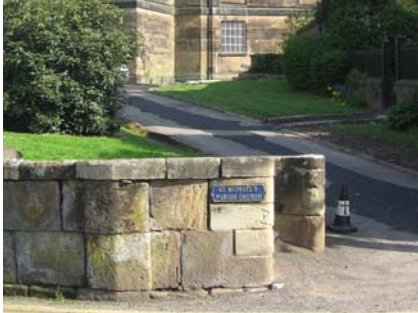
I4a Ashlar stone boundary wall
